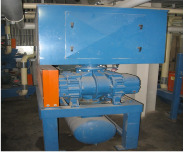
Typical Positive Displacement Blower
